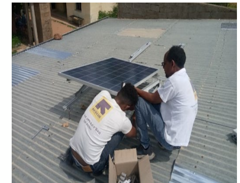
Installing solar panels, Ethiopia
